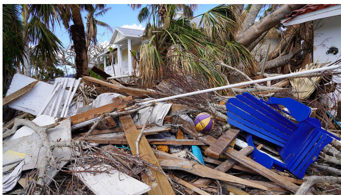
Houses along the shoreline are destroyed by Hurricane Ian in Florida.
